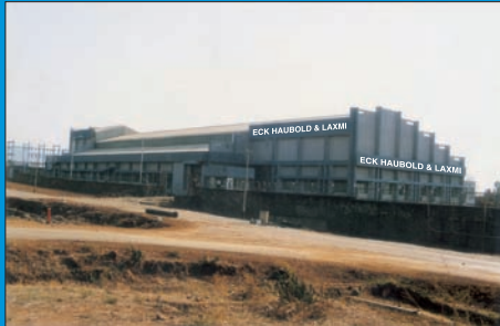
Manufacturing Plant at Ambarnath
